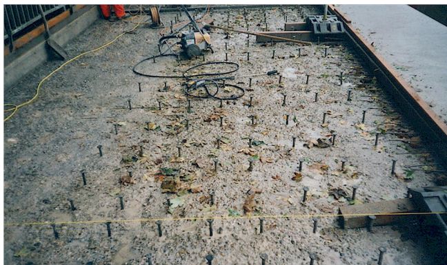
Brückensanierung in Olten Bridge renovation in Olten
