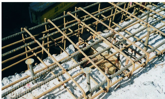
Brückensanierung in Riddes VS Bridge renovation in Riddes VS
